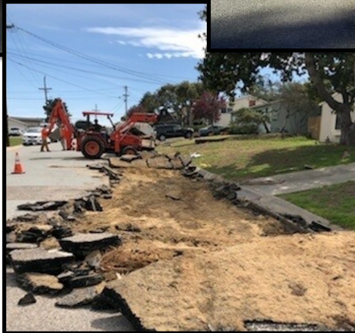
Above and to the right: Public Works digging up and repairing tree root damaged streets in preparation for the slurry seal project starting in June. They are using the tractor purchased with grant funds.
