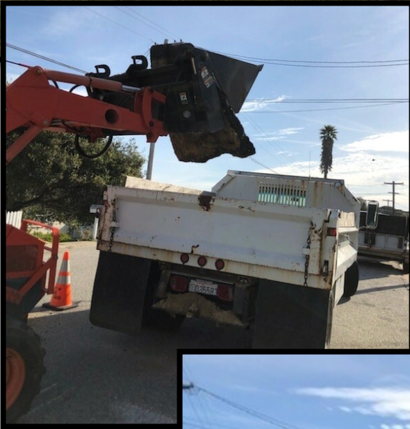
Above and to the right: Public Works digging up and repairing tree root damaged streets in preparation for the slurry seal project starting in June. They are using the tractor purchased with grant funds.
